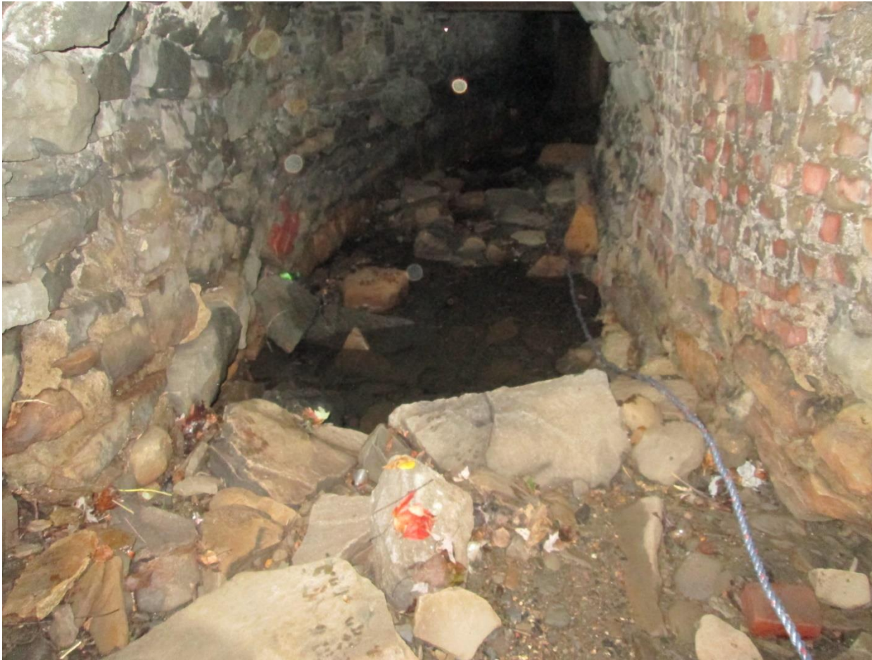
Existing culvert near Delaware Street
