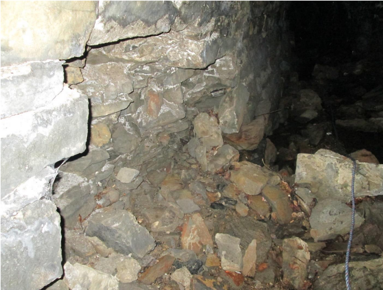
Existing culvert near Delaware Street
