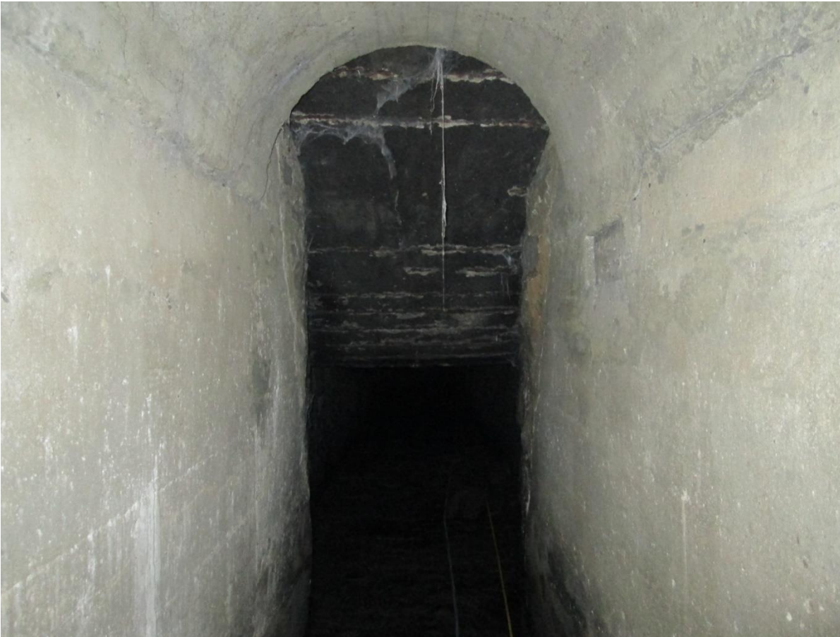
Existing culvert under Washington Avenue/Sturgis Park
