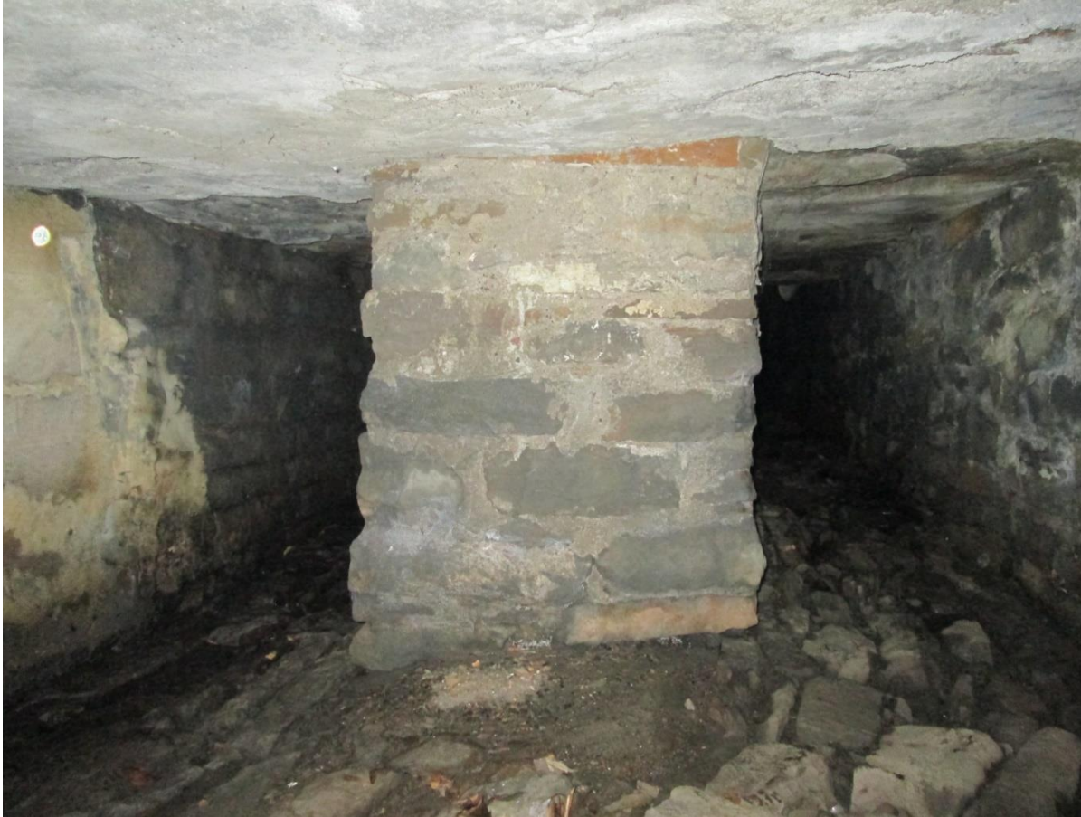
Existing culvert under Electric Street
