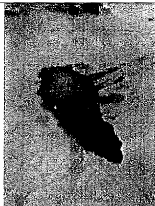
Photo #12: Localized oil staining seen in garage - REC.
