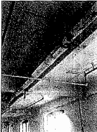
Photo #13: Suspect asbestos containing pipe insulation
