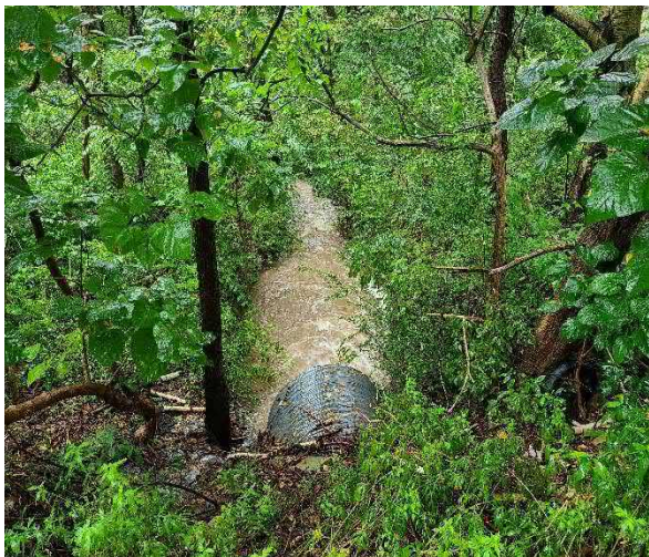
Figure 24 - 48" CMP to Dry Dam @ 2pm
