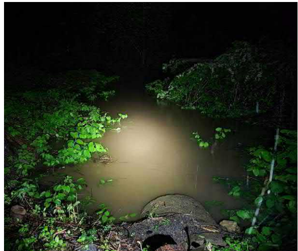
Figure 5 - Keyser Creek Outfall Showing Tailwater Condition @ 8pm
