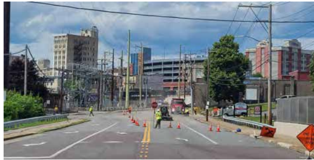
View north from Cedar Avenue Bridge
