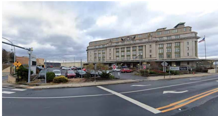
The parking lot enfronting the former train station
