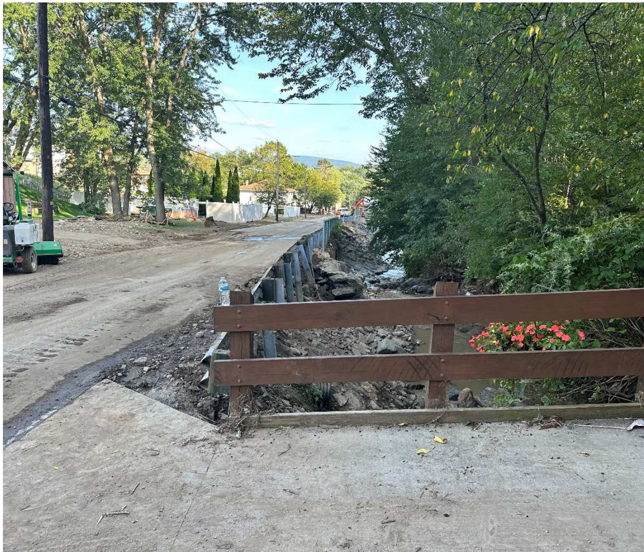
Lindy Creek, Looking Downstream
