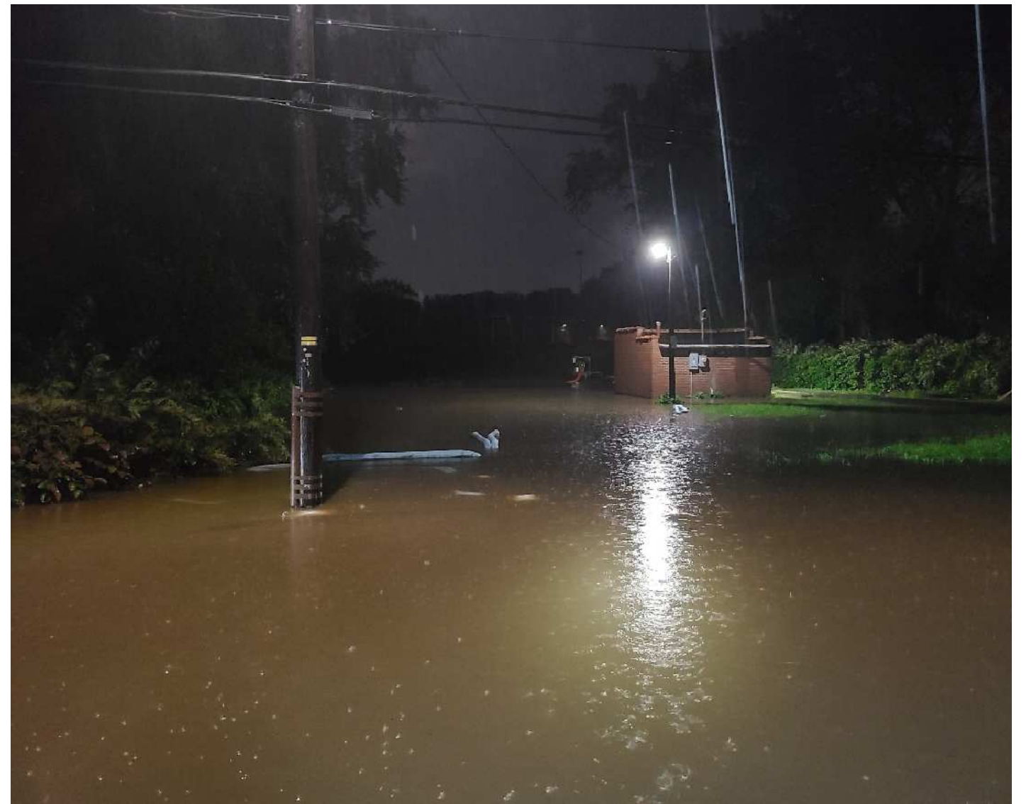
Merrifield Pump Station, 8pm
